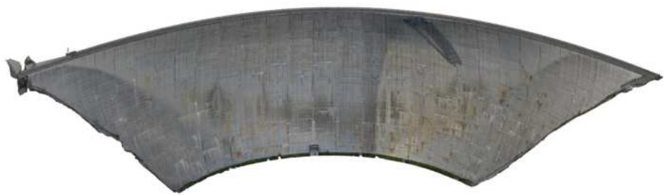
High resolution dam geometry from operator (drone survey)
