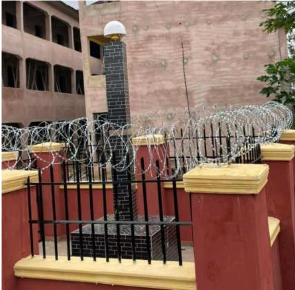
Figure 4: SOGPOS Abakaliki CORS Monument (Tersus AX3707 Choke Ring Antenna)
