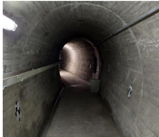
Figure 1: Conditions inside the gallery of the arch-gravity dam
