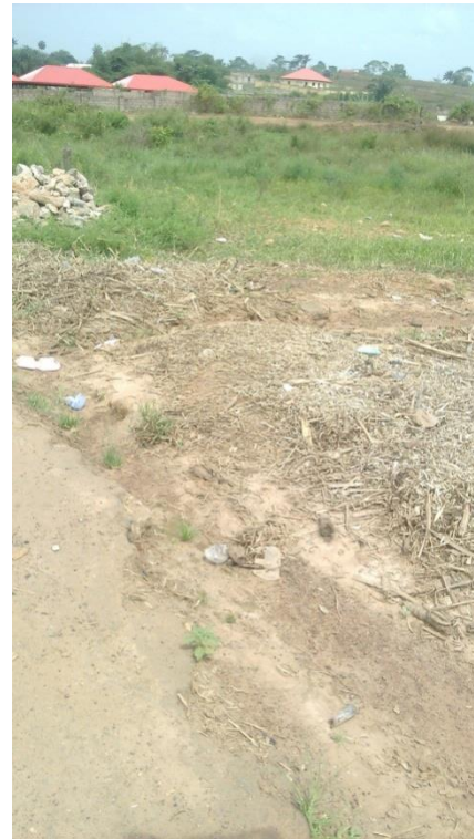
Figure 12: Impact of Reclamation on Infrastructure (Drainage 2018)
