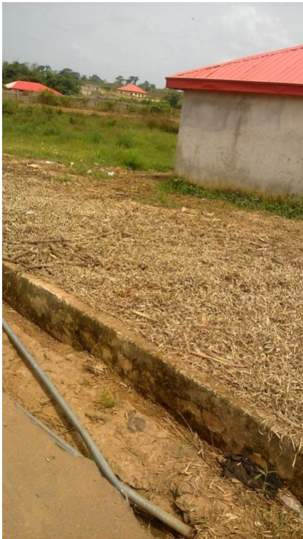
Figure 11: Impact of Reclamation on Infrastructure (Drainage 2018)
