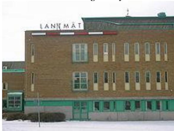
Figure 9. The Real Property Register stands for a stable and secure real property market.
