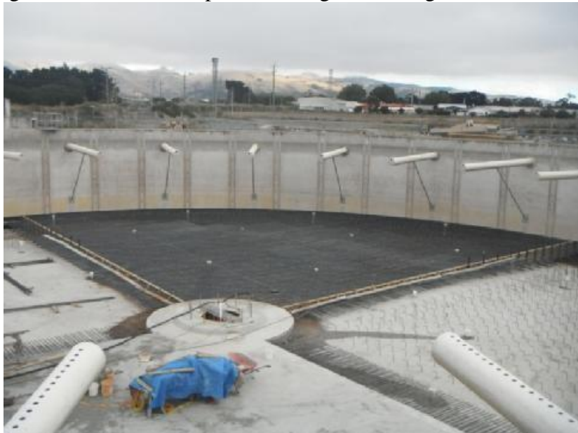
Figure 12: Clarifier 3 repairs showing reinforcing mats
