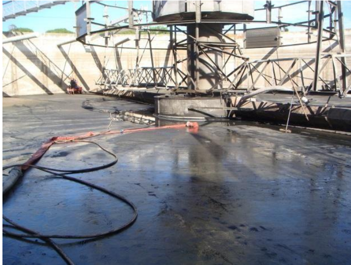
Figure 5: Clean Out of Clarifier 2
