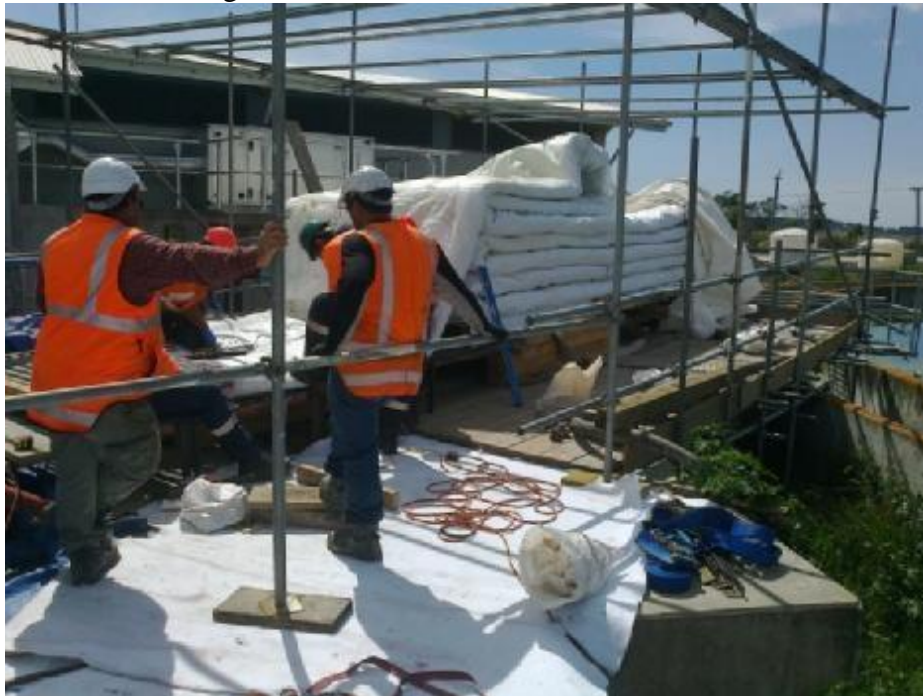
Figure 10: CIPP Liner Prior to Installation
