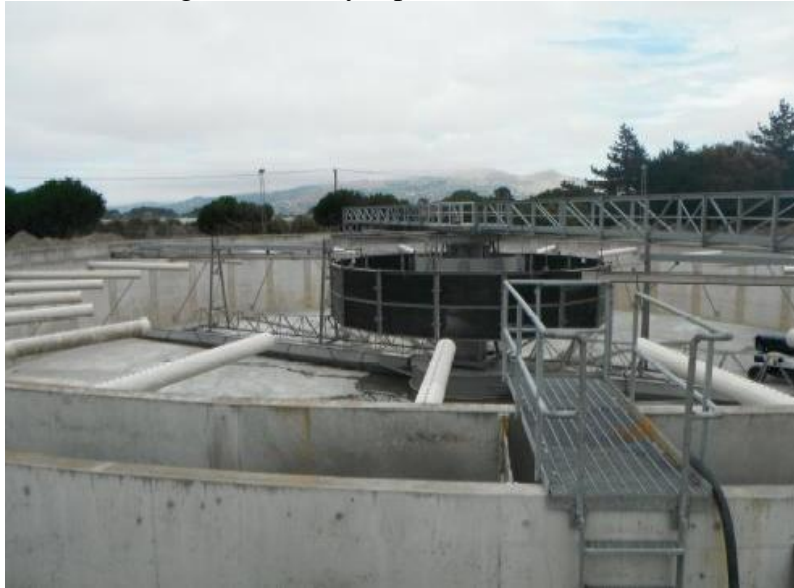
Figure 13: Fully repaired Clarifier 4
