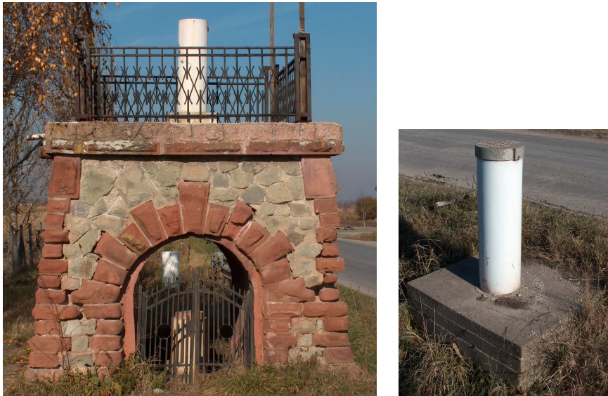
Fig. 11: Reconstructed end point of the Paraćin basis and one of the pillars
