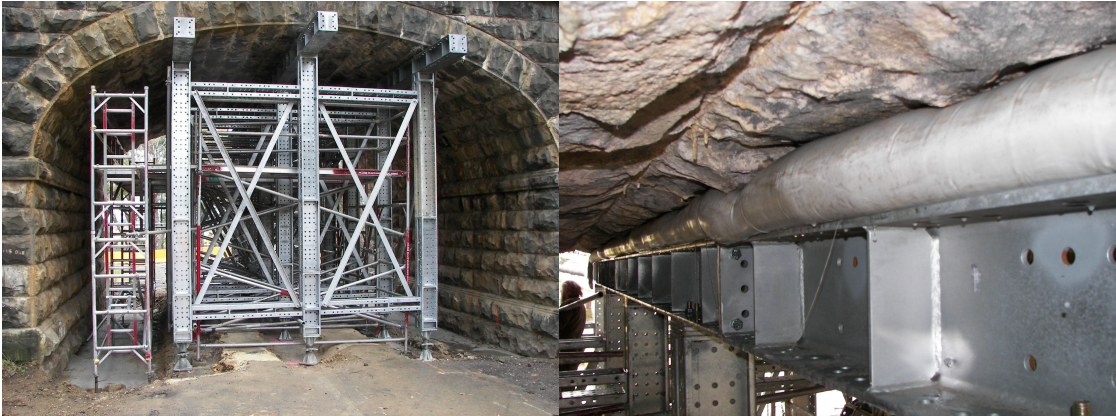
Fig 13: Propping using proprietary false-work and grout bags.
