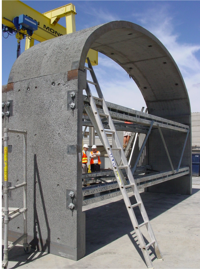
Fig 15: Trial assembly of the precast concrete liner.
