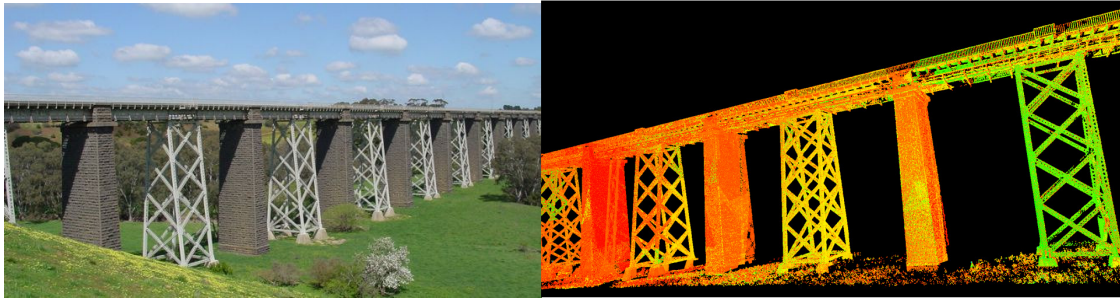
Fig 2: Moorabool Viaduct image and laser scan point cloud.
