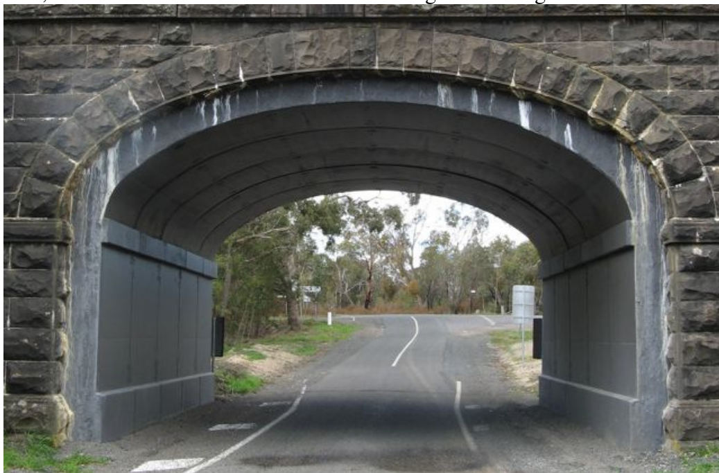
Fig 17: Completed strengthening works.
