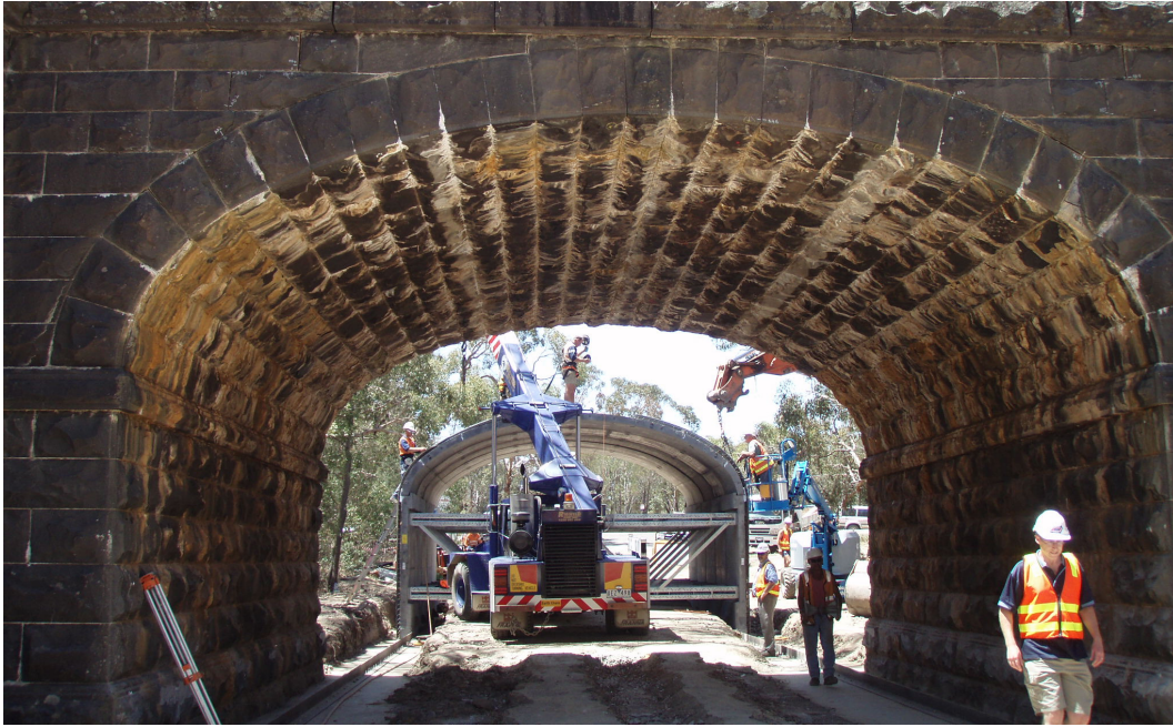
Figure 16: Precast concrete liner ready for sliding (with reo attached).
