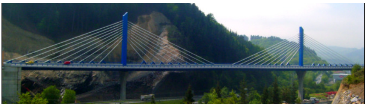
Lateral view of Arbizelai's bridge
