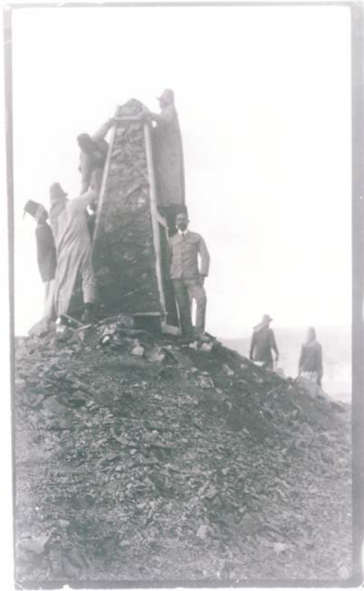
Fig 3: The Construction of the (Parker) Pillar at Taba on 31 December 1906
