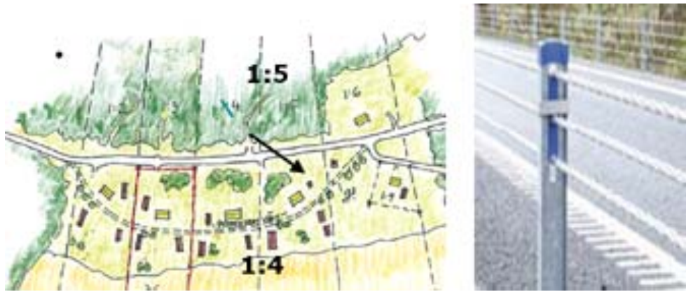
Figure 4: A cable barrier
