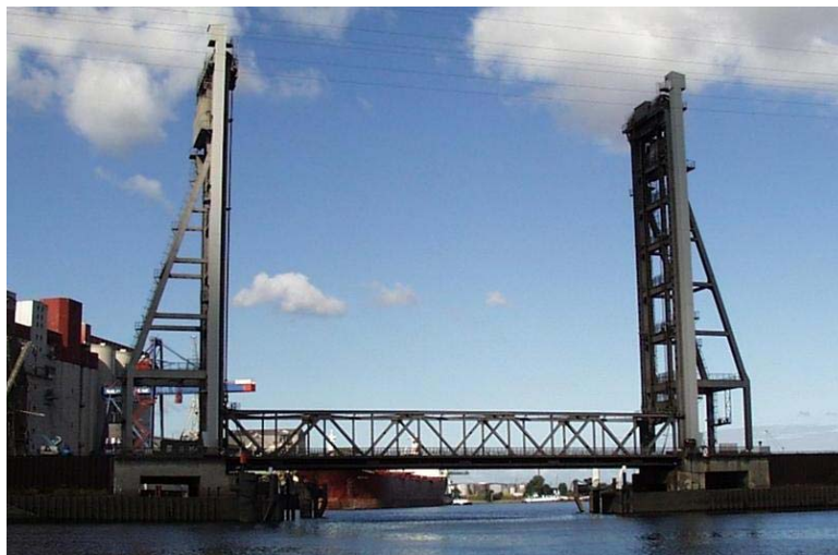
Fig.1: The Rethe vertical lift bridge while road and rail traffic crossing the bridge
