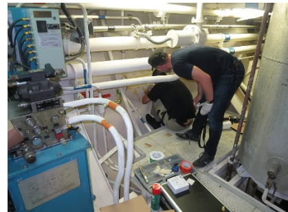
Figure 4. Gluing of the FBG sensors in the engine room
