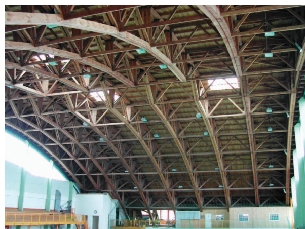
Figure 3 Roof after its completion
