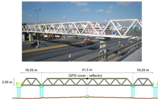
Figure 1. View of the pedestrian footbridge crossing the Kifisos Avenue in Athens (up) and location of the sensors used to measure the bridge oscillations (down).
