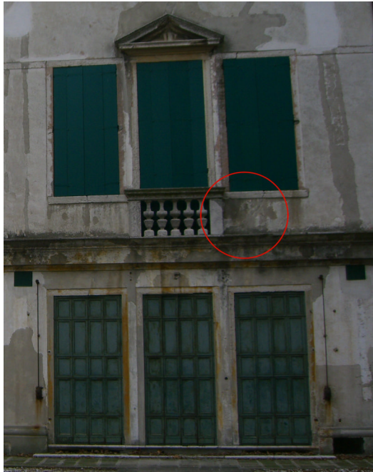
Figure 3: Partial view of the east wall
