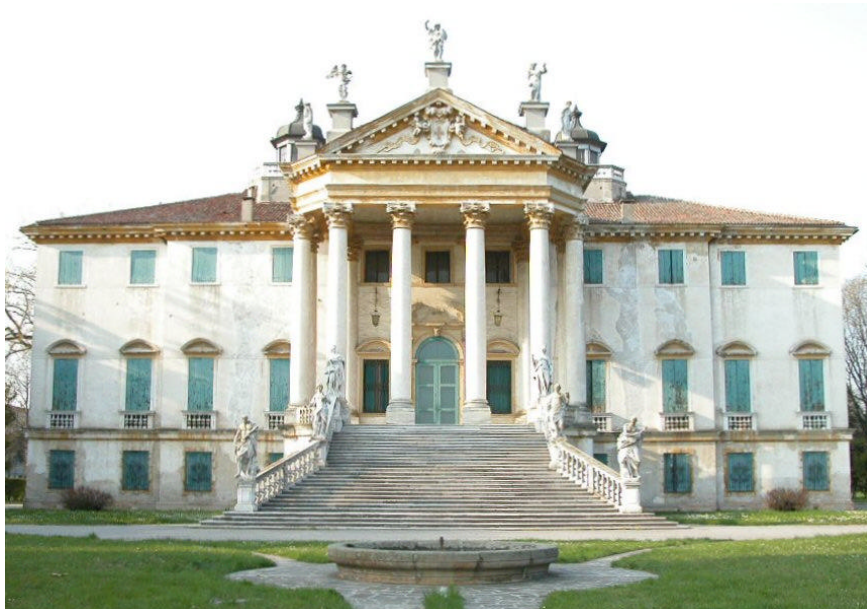
Figure 1: View of the front side of Villa Giovanelli
