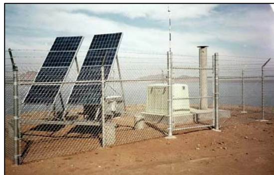
Figure 2. CGPS site at the East Dam
