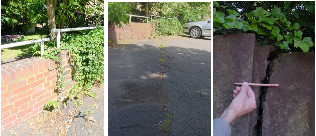
Figure 3: A special section of the Erft Fault, called Donatussprung, can be easily identified at the surface.
