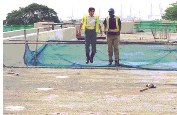
Figure 10: Pasir Panjang Semi-expressway under construction
