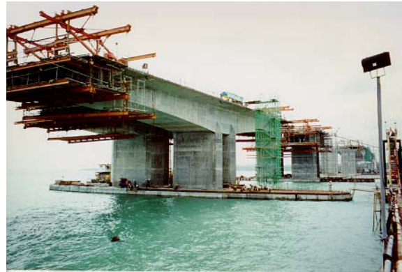
F Figure 1: Tuas Second Link bridge under construction
