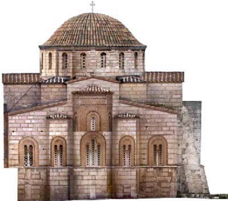
(a) Orthophoto-mosaic of the eastern external façade of the church
